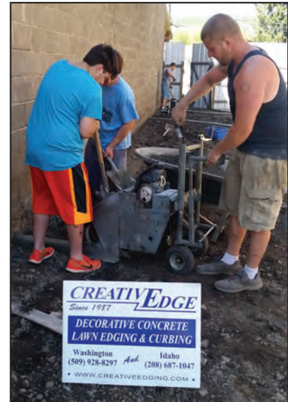
Ground preparation; then edging.
